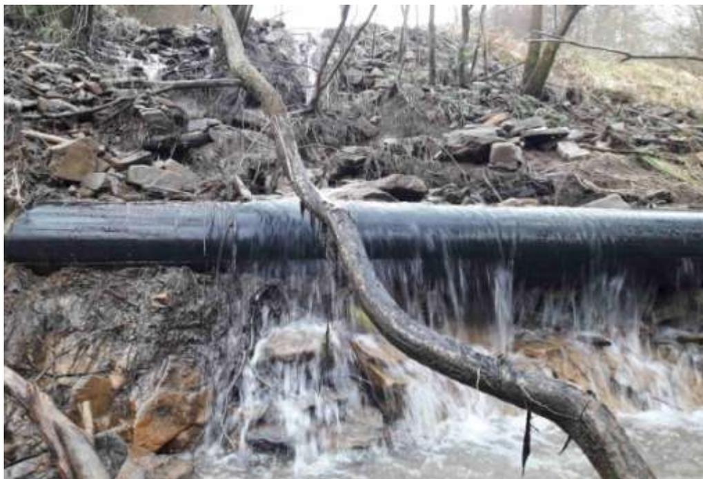
Photo: Exposed penstock pipe at Cwm Saerbren following the landslip in early March
