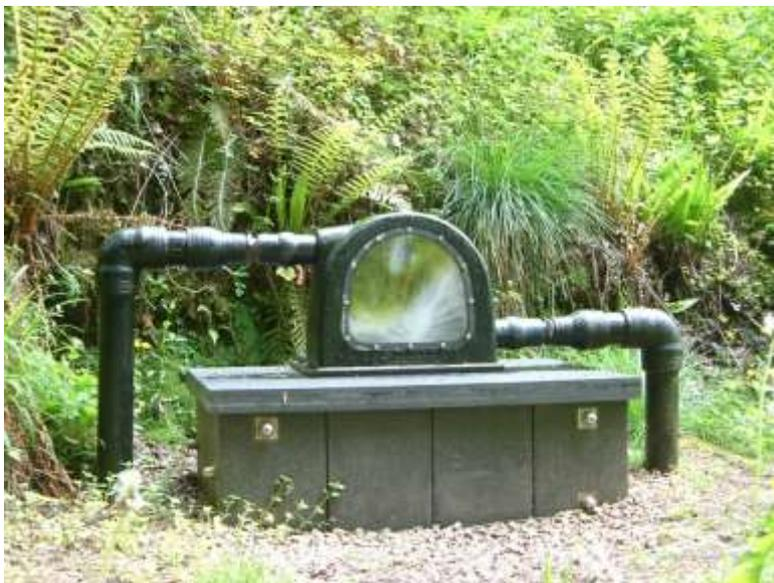
Running since autumn 2013, my Powerspout Pelton runs all year, even in the driest months. Its max output is 920 W (22 kWh /day) going down to 100 W at the driest times. With 3.2kWp of solar installed on a barn roof, it has meant our take from the grid is only about 2000 kWh per year; for a house which is electric only (+ wood heating) and a Nissan Leaf car, I'm well pleased we're doing our bit to save the planet.
