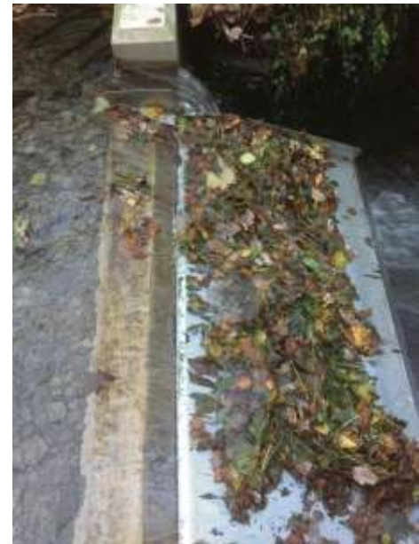
Image: Abernant intake last month – before cleaning!
