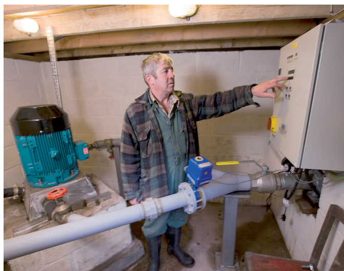
Inside a typical turbine house, with, from left to right, the turbine housing, generator, pipework and switch gear
