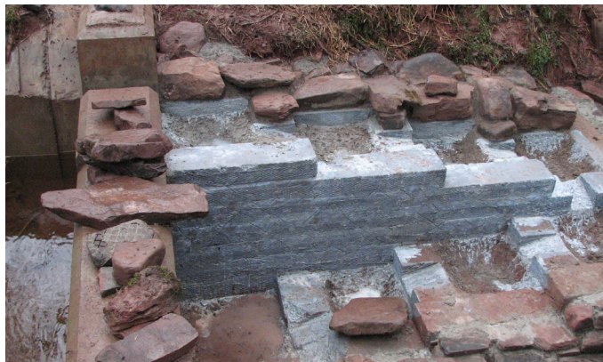
A typical intake with fish pass during construction
