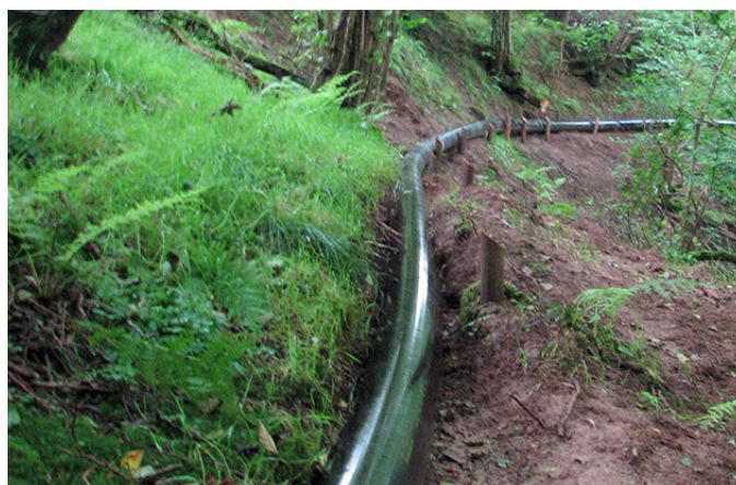
Penstock is surface laid in woodlands to minimise damage to tree roots and is soon obscured by vegetation
