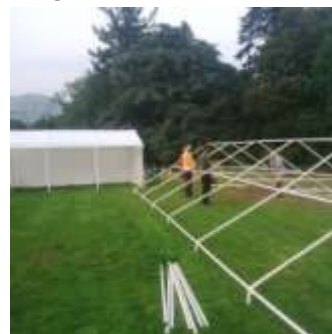
Marquee construction before the show
